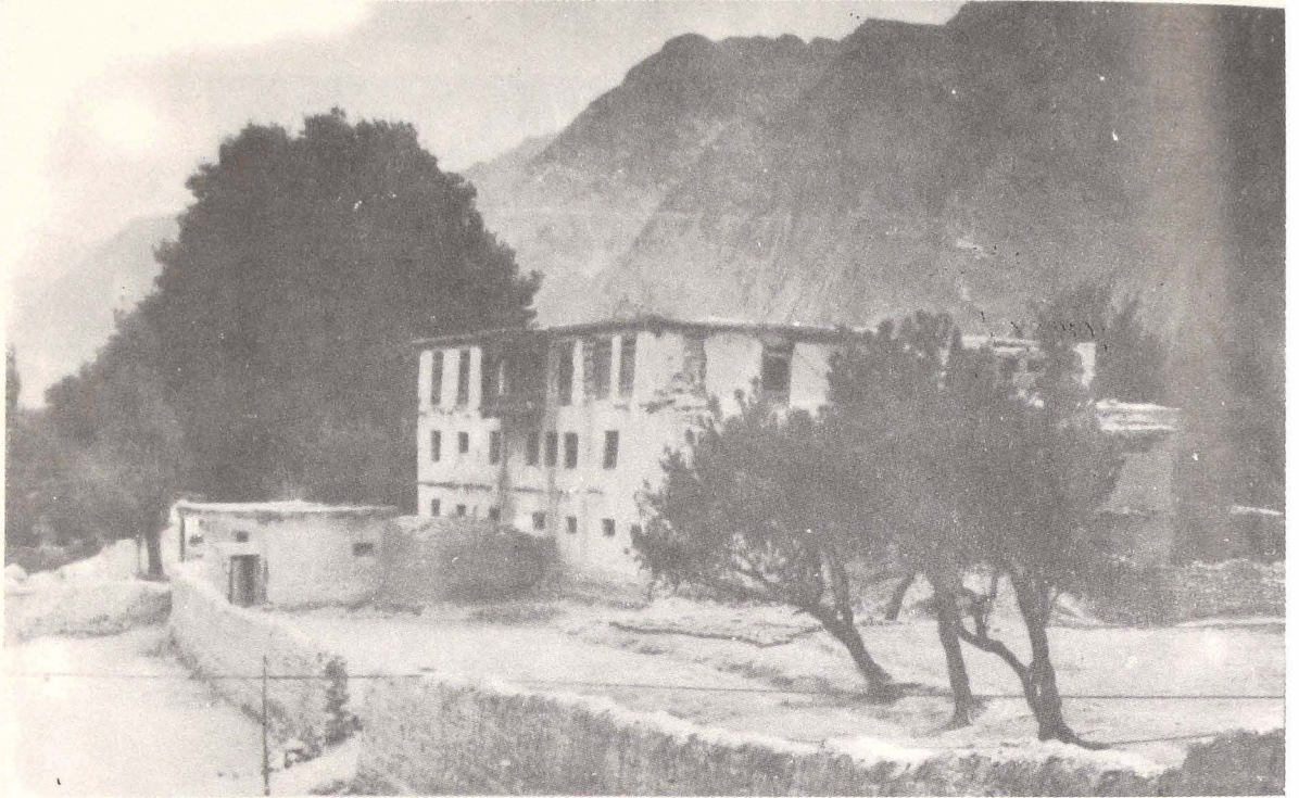
Pl. 35. Skardu — Raja's Palace, renovated in modern time.
